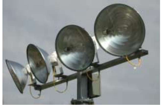
Figure 27 - Top-mount Tubular Cross Arm
