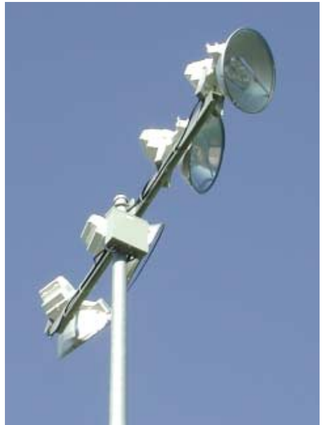
Figure 28 - Side-mount Angle Cross Arm
