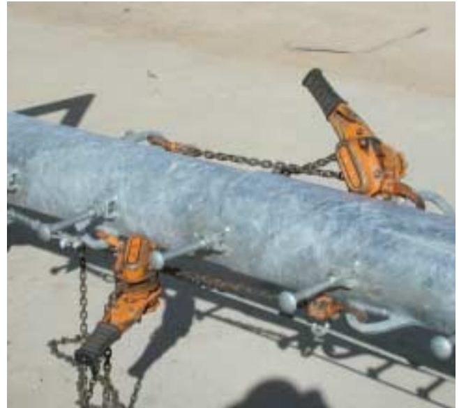
Figure 10 - Slip Joint Assembly
