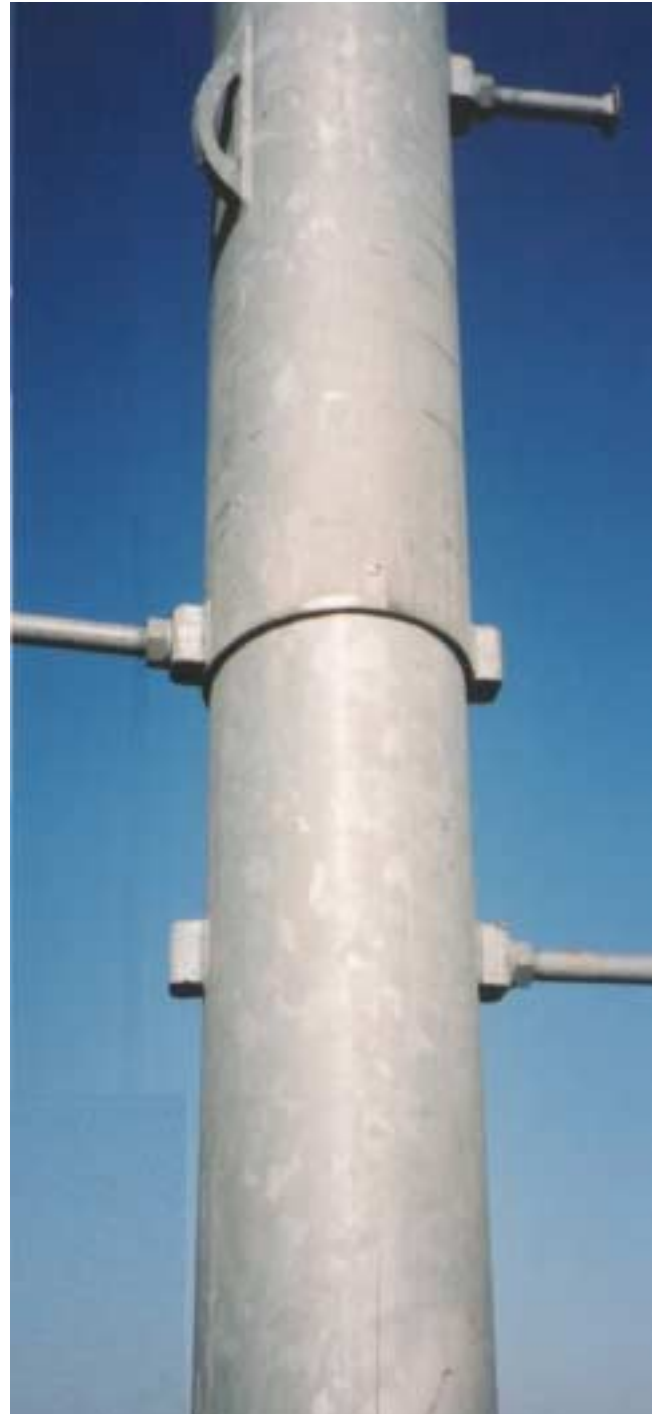
Figure 7 - Proper Slip Joint
