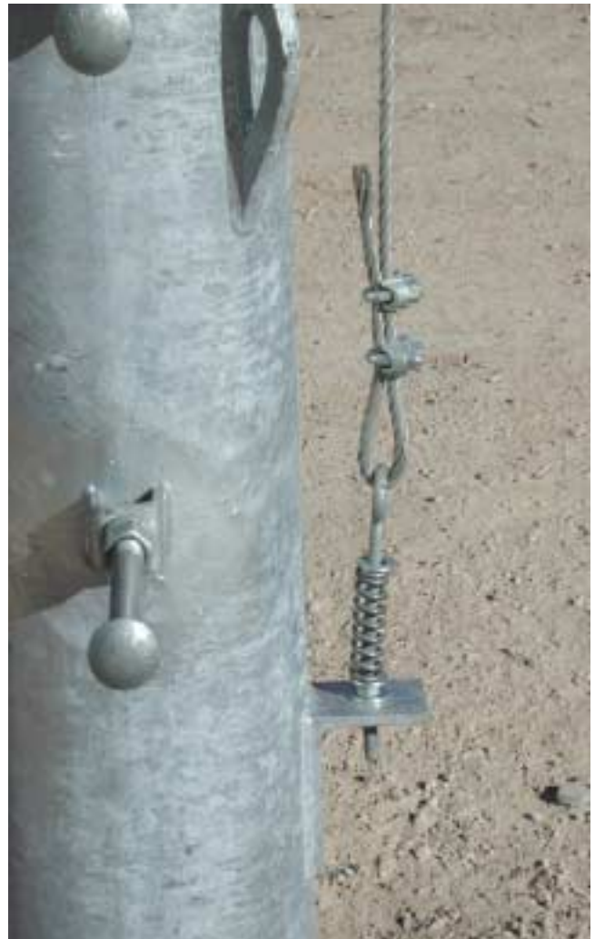
Figure 14 - Bottom Cable Stop (CAB-STP-B1)
